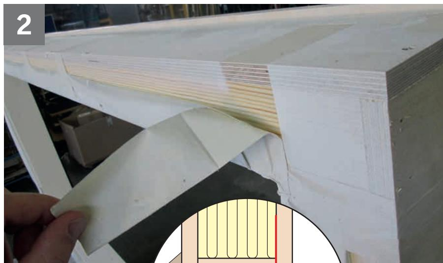
**ENGLISH:** Remove the tape from the bottom of the frame to release the vapour barrier. Allow the vapour barrier to suspend in the hole.
